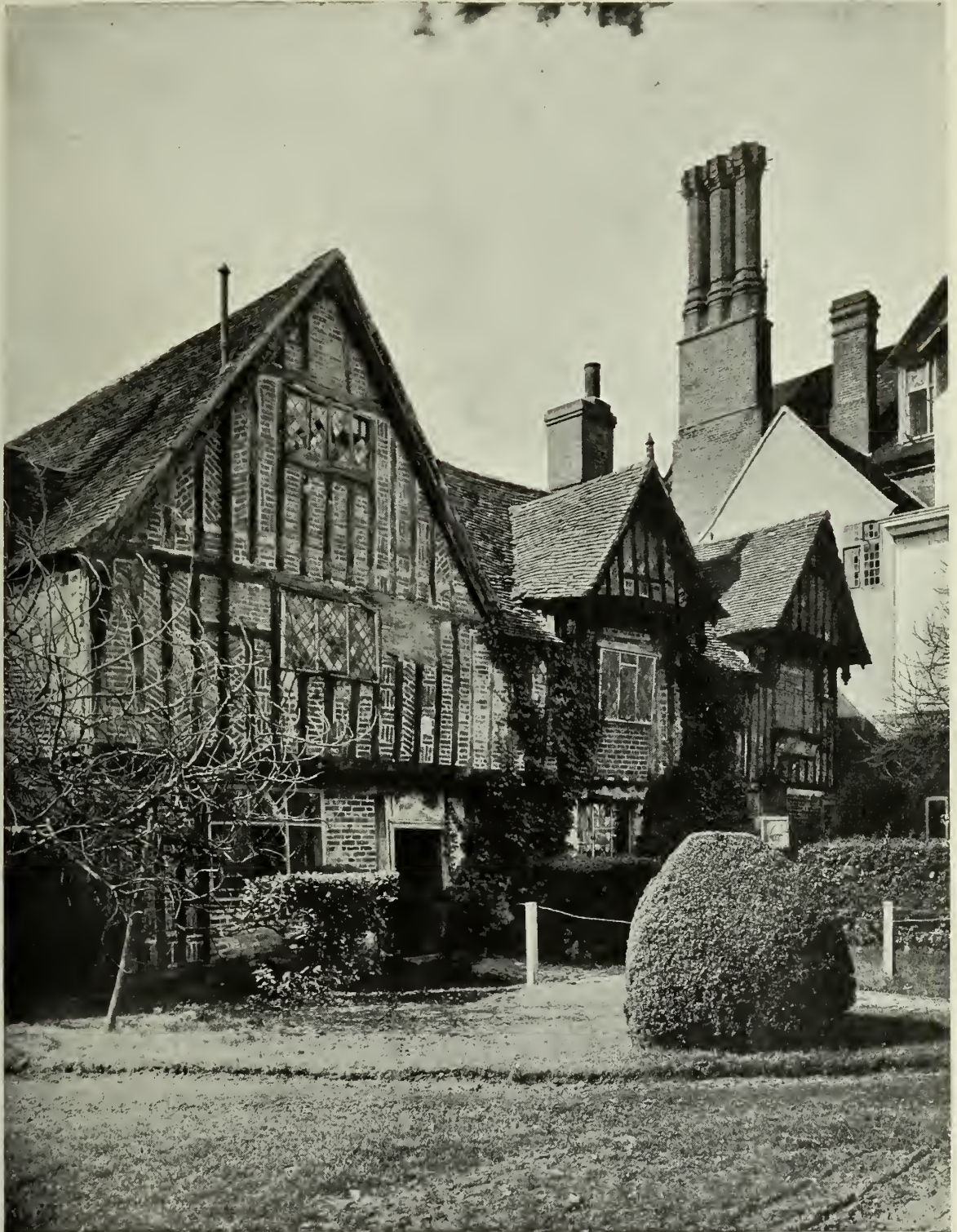
STEEPLE BUMPSTEAD : MOYNS PARK. South-West Wing ; early 16th-century.
